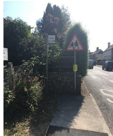
Photograph 6: Termination of Footway at Bus Stop
