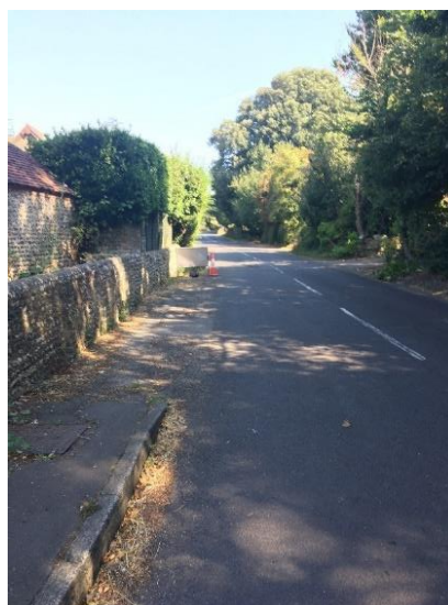
Photograph 1: Tye Lane Footway
