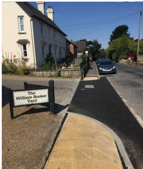
Photograph 9: Crossing facility at The Street/William Booker Yard Junction
