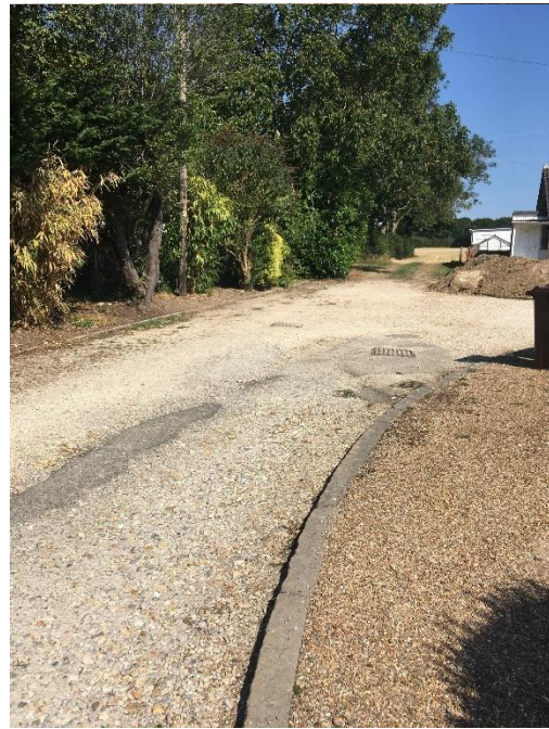
Photograph 15: Field Close connection to Site
