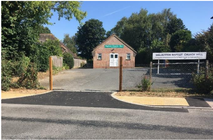
Photograph 5: Crossing Facility Outside Baptist Church
